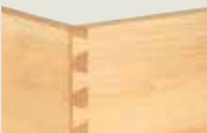
Partially covered dovetail joints
