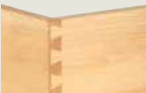
Partially covered dovetail joints
