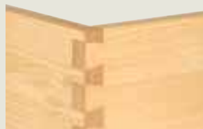
Open dovetail joints
